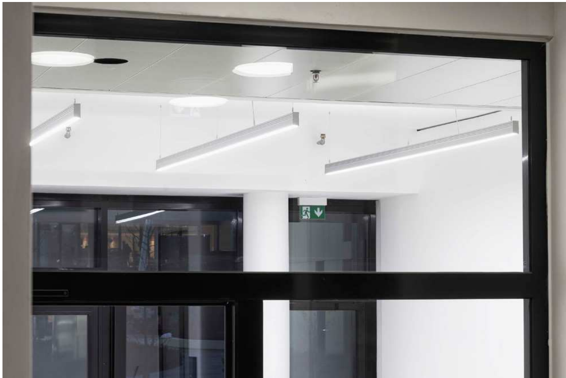
Filligree shape and homogeneous light: The pendant luminaire “LED Linargo” offers indirect light up and direct light down. At night, the luminaire switches to indirect light. Photo © ADO Lights by TTC Timmler Technology GmbH / photographer Peter von Pigage
